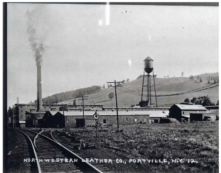
Another view of the Northwestern Leather Co. looking toward "Bear's Cave". In the foreground is the Pittsburg, Shawmut and Northern Railroad tracks and the siding that went to the tannery
